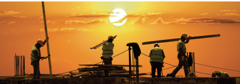
Roofers are subject to triple digit temperatures.
